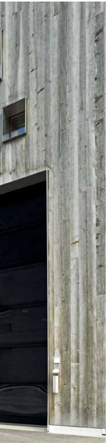
TOP. ALR F42 with on-site flush-fitting cladding made of aluminium compound boards
